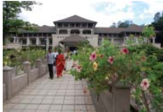
Kandy Court Complex – Automated in 2006
